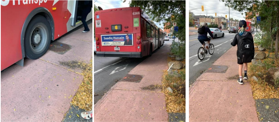
Figure 04, 05 & 06 – Bus turning right from Acacia onto Beechwood and mounting the curb due to the tight turn.
