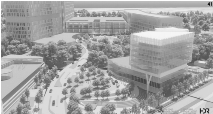
Photo: Digital rendering of the Ottawa Hospital's new Civic Campus. (credit – TOH)
